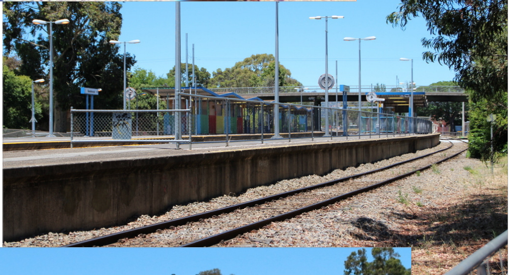
Standard gauge line running behind platform 3
