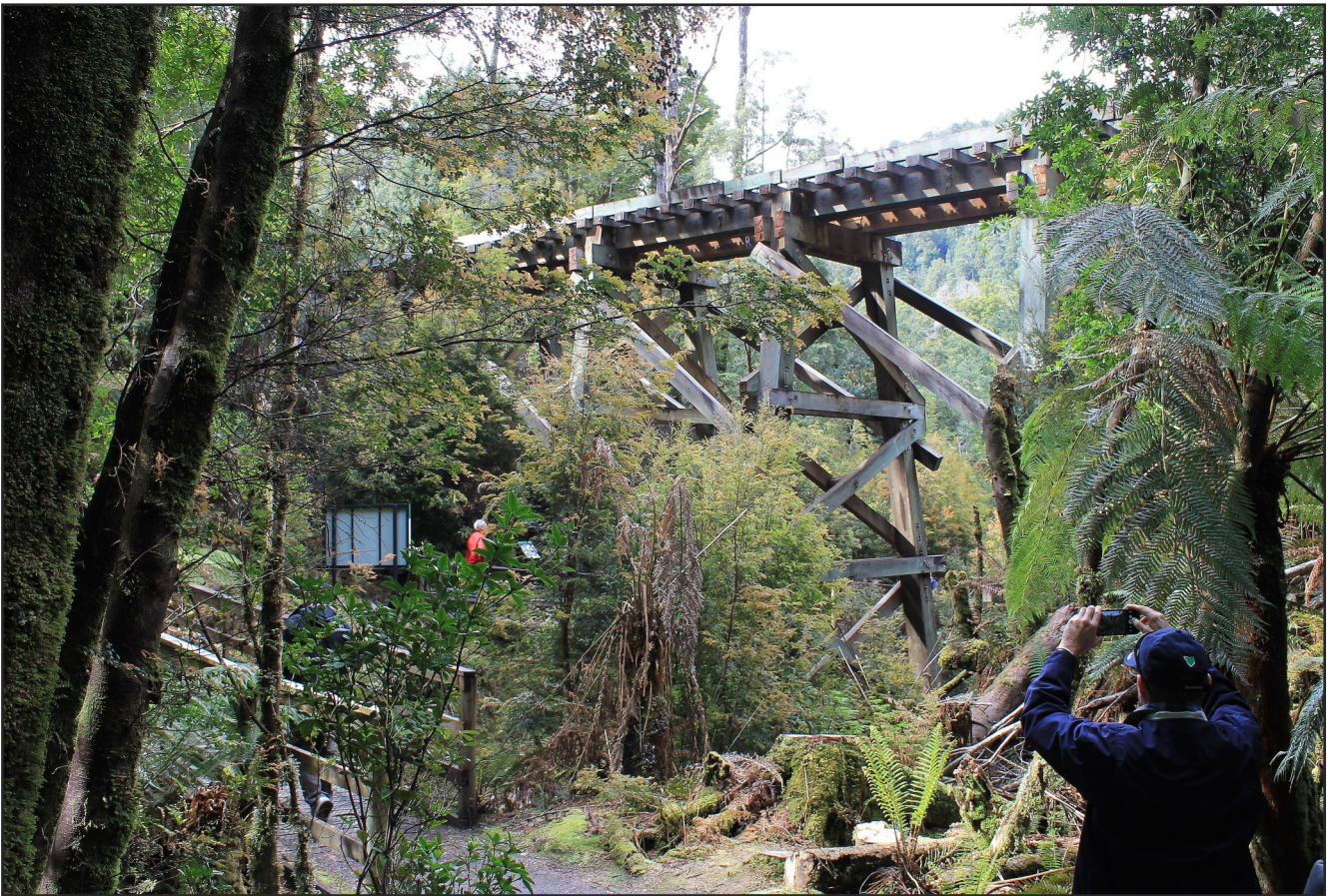
Trestle near Dubbil Barril
