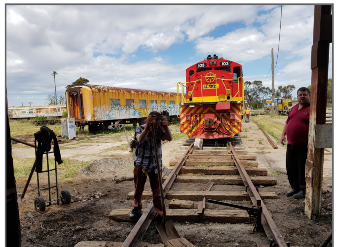
Track laying crew - SARMA members hard at work getting the track into the shed sorted.
