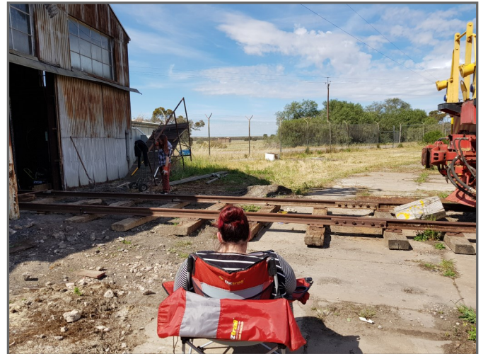
Foreman Watches - Sherree takes a break while Dane lays the dog spikes into the new section of track
