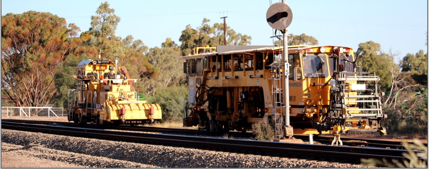
Track machines at Crystal Brook working on newly installed switch
