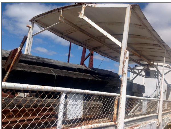
Photo 15. RH stanchion construction. Note also small diagonal piece on LH stanchion opposite. 01.01.2017.
