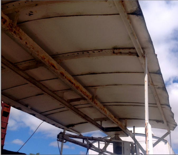
Photo 19. Crane Runway detail. 01.01.2017. Taillem Bend. Author photo.
