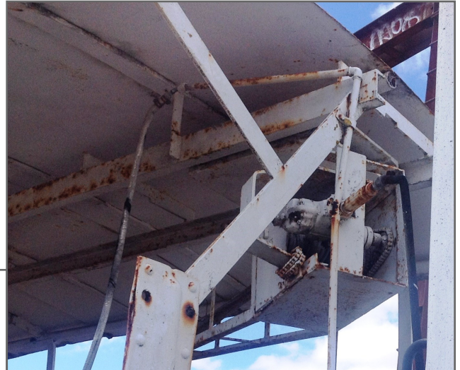
Photo 24 (right): Crane motor detail. 01.01.2017. Taillem Bend. Author photo.
